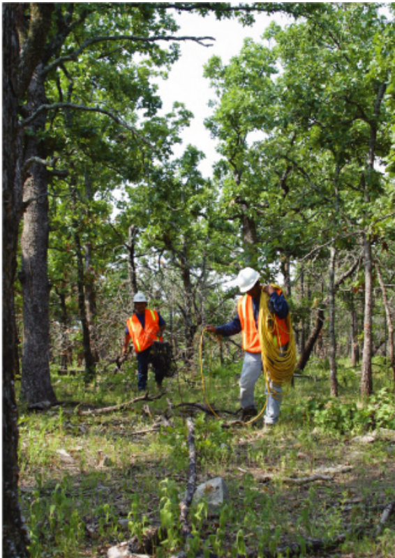
Crew deploying geophones and cables.
